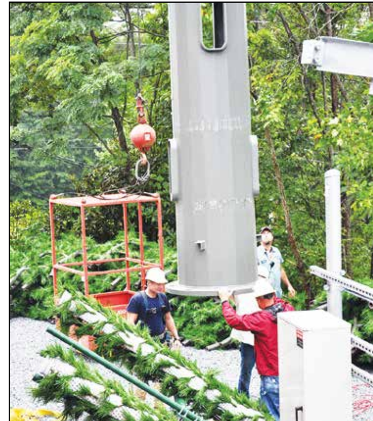
Workers secure the base to the pad.
