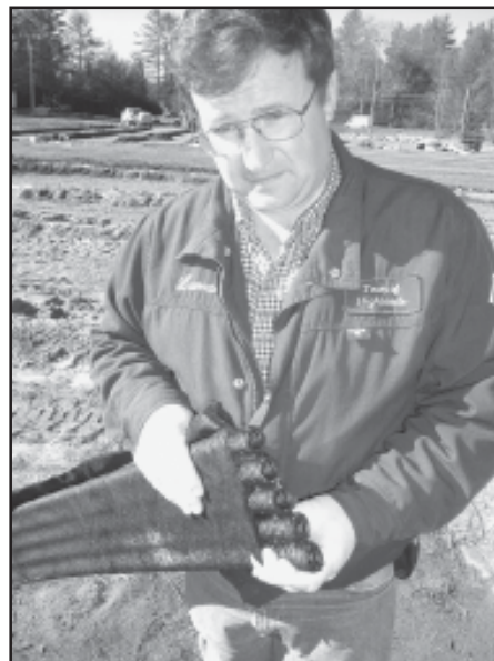
Town Engineer Lamar Nix hold the multi-flow piping which is being set on edge in scores of ditches across the baseball field.
