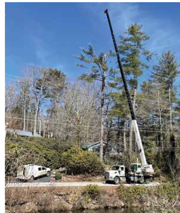
Crews near Riverwalk and Mirror Lake. Photo by Capt. Leah McCall
