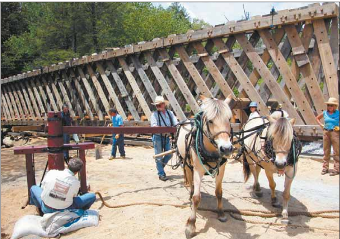
Using a winch system alternately powered by horses and oxen, the bridge at The Bascom site on Oak Lane slowly inched its way across the creek to form the bridged entrance to the gallery's site. Joe Luke and his team take a turn.
