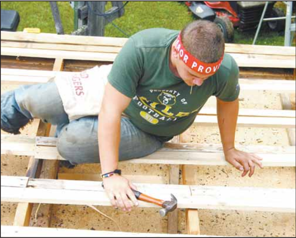
Above, Alex Robinson works on the roof of the main house. First old, rotten shingles were removed and then a new roof installed. The group also re-tinned the back porch roof, cool-sealed the front porch roof and painted the porch hand rail.
