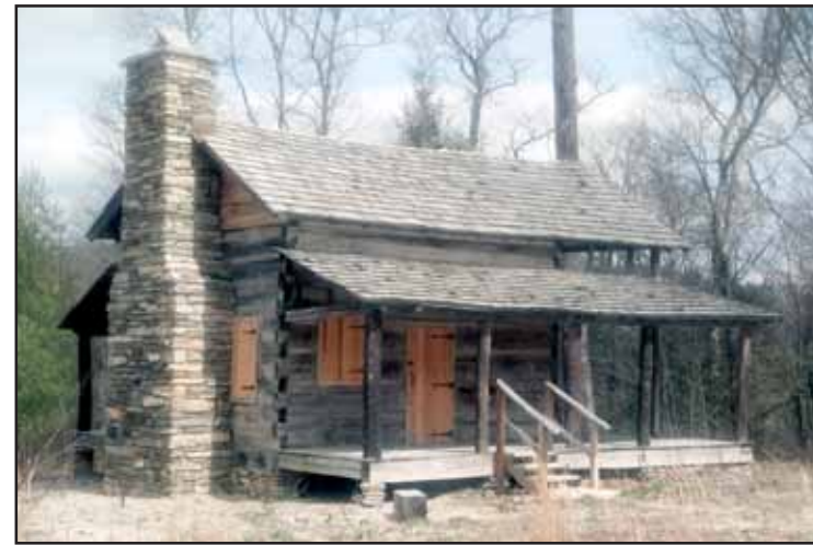
Slowly, the McCall cabin is being renovated for use.
