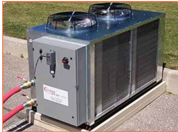
Above from left: tubing through which glycol is pumped, the rink lined with plastic tubing and filled with water, and the 4,000-lb. chiller machine.
