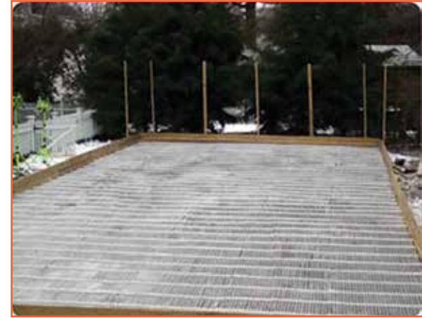
Above from left: tubing through which glycol is pumped, the rink lined with plastic tubing and filled with water, and the 4,000-lb. chiller machine.
