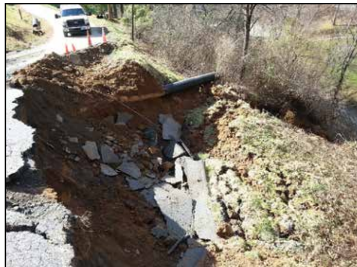
This is a shot of a driveway that failed and fell into a stream below during the early December 2015 rains.
