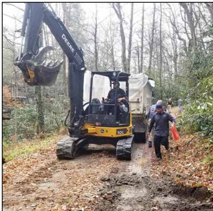
Contaminated dirt will be taken to a Subtitle Landfill for disposal. Absorption pads will be replaced at least twice a day at the point of egress.
