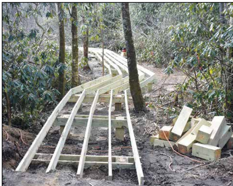
Above: HBS Project Coordinator Sonya Carpenter said they are taking all precautions possible to protect the environment throughout the construction process, including using a crane to pound in the pylons to avoid bringing heavy machinery into the wetland.
