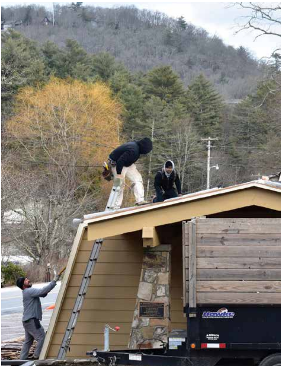
Roofers removing old shingles on the Community Building on Poplar Street.
