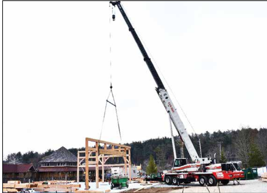
The framer on the lift gives the crane operator hand signals to tweak the beam's position to fit the oak pin into the beam. Crews from Moresun Timber Frames used two cranes to manipulate the beams into position. All the beams and jointery were hand cut.
