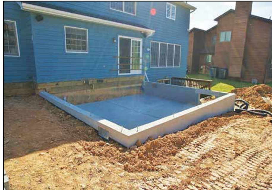
Foundation for ground floor addition.
