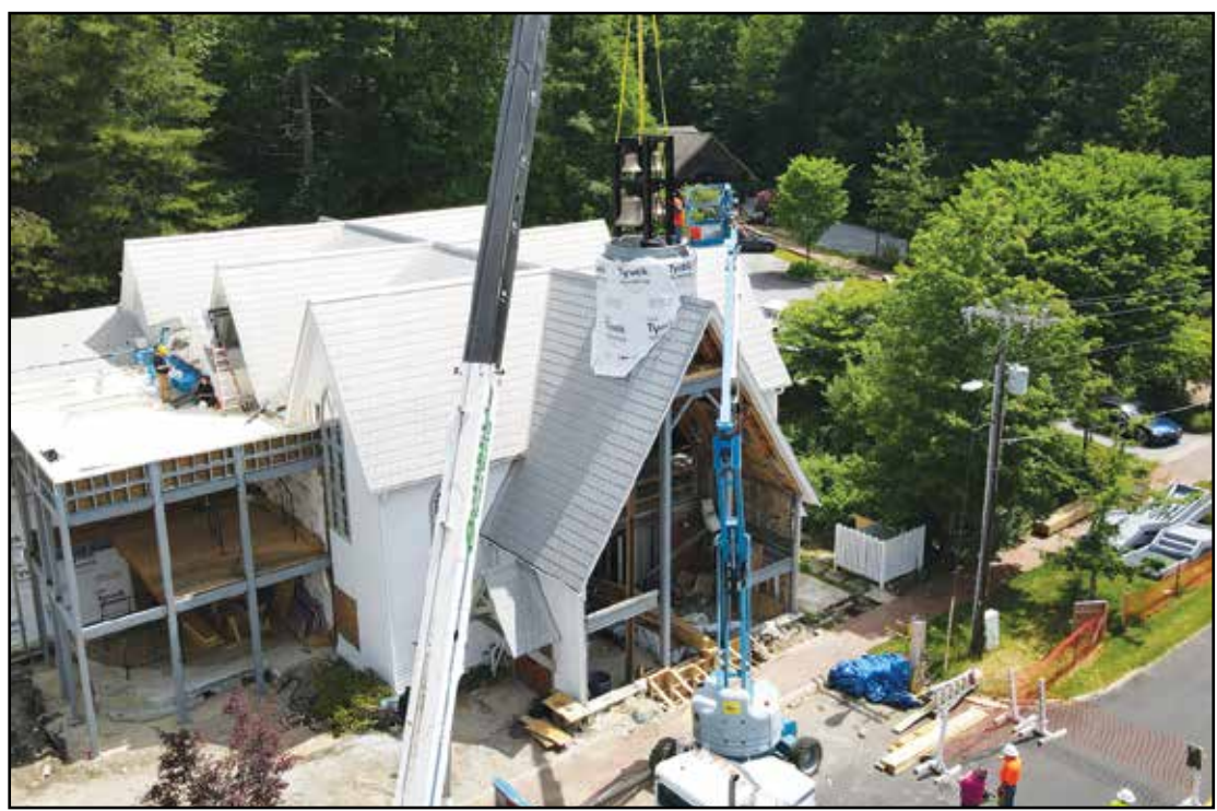
A crane hoists 4,500 lbs. of bronze bells onto the spire of the Episcopal Church of the Incarnation at 5th and Main streets. — Photo by Brian O'Shea
