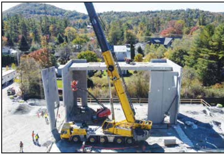
Pre-cast concrete walls for the 300-seat theater are going up. – Photo by Brian O'Shea
