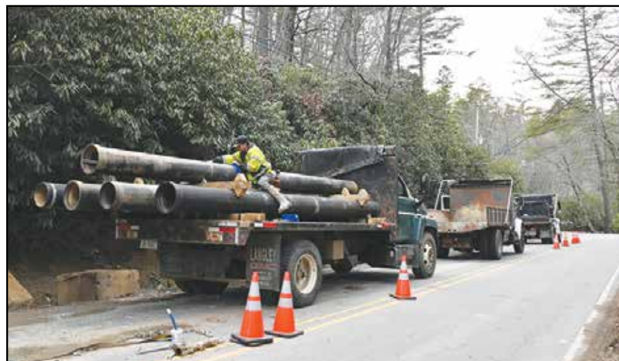
Crews made permanent repairs using materials the town had on hand – 12-inch Ductile Iron Pipe - which is the same as the original pipe. The town is preparing a study of the line to determine if any other areas need to be replaced while considering other materials for longer range alternatives.
