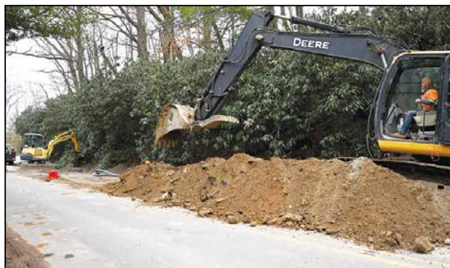
Workers started to repair the line as soon as the W/S dept. noticed it on Wednesday of last week. A substantial section of the 29-year-old sewer pipe had failed due to deterioration which caused numerous breaks in the line.
